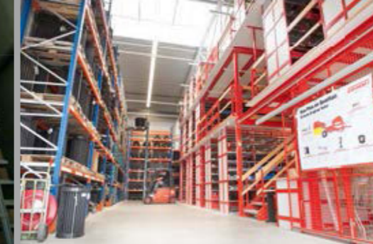
Warehouse at Grimme Uelzen Modern storage and warehouse-systems at the plants of our subsidiaries and the Grimme Premium Partners ensure the supply of all spare parts.
