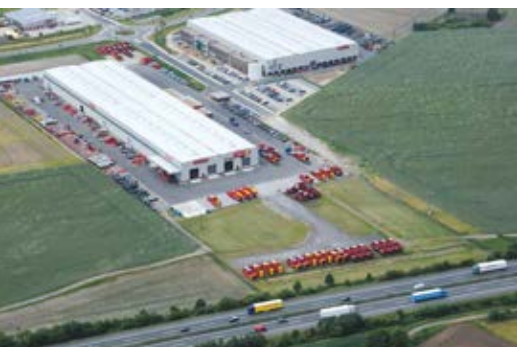
Factory 2 in Niedersachsenpark, 12 km away from the headquarters
